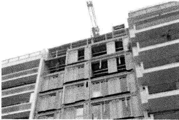
photo North by NorthWest Architectes
